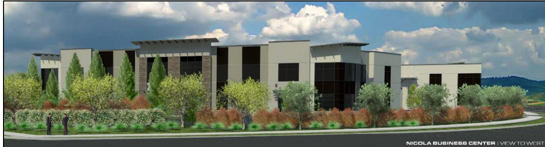
View from Fremont Connector / Nicola Avenue Intersection
